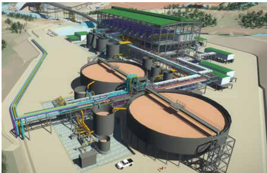
A Turnkey Dry Stacking Tailings Facility (thickening, pressure filtration, conveying, stacking)
